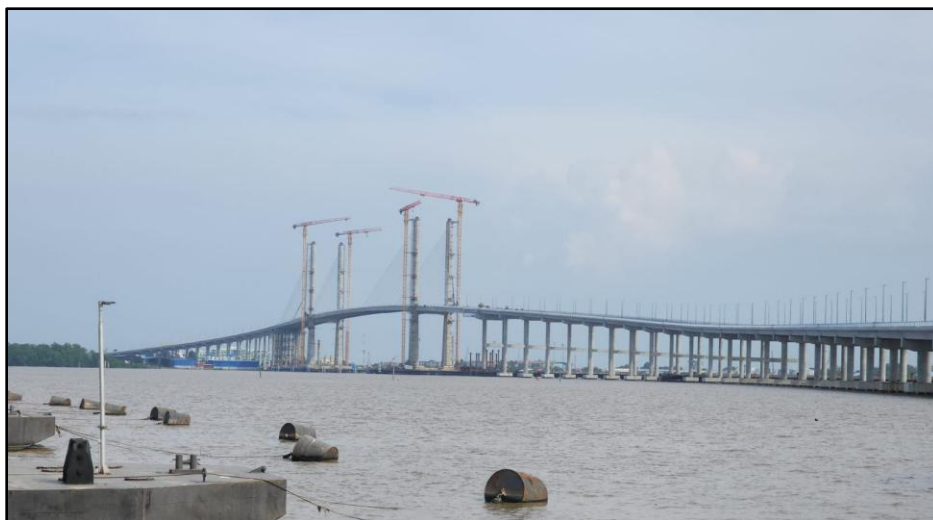
Photos of the New Demerara River Bridge- 18 September 2025
