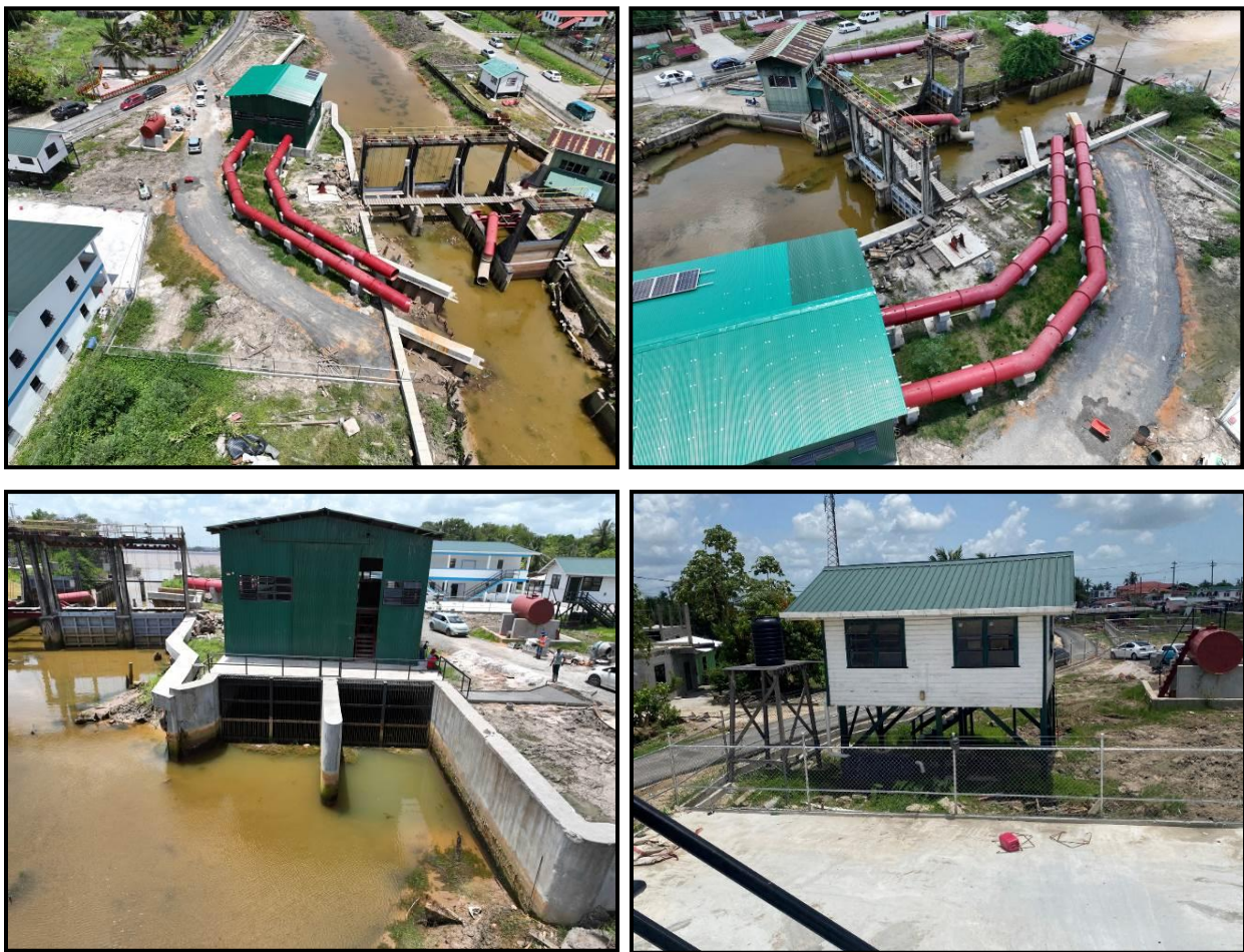
Photographs of Canal №.1 Pump Station - 22 August 2024
