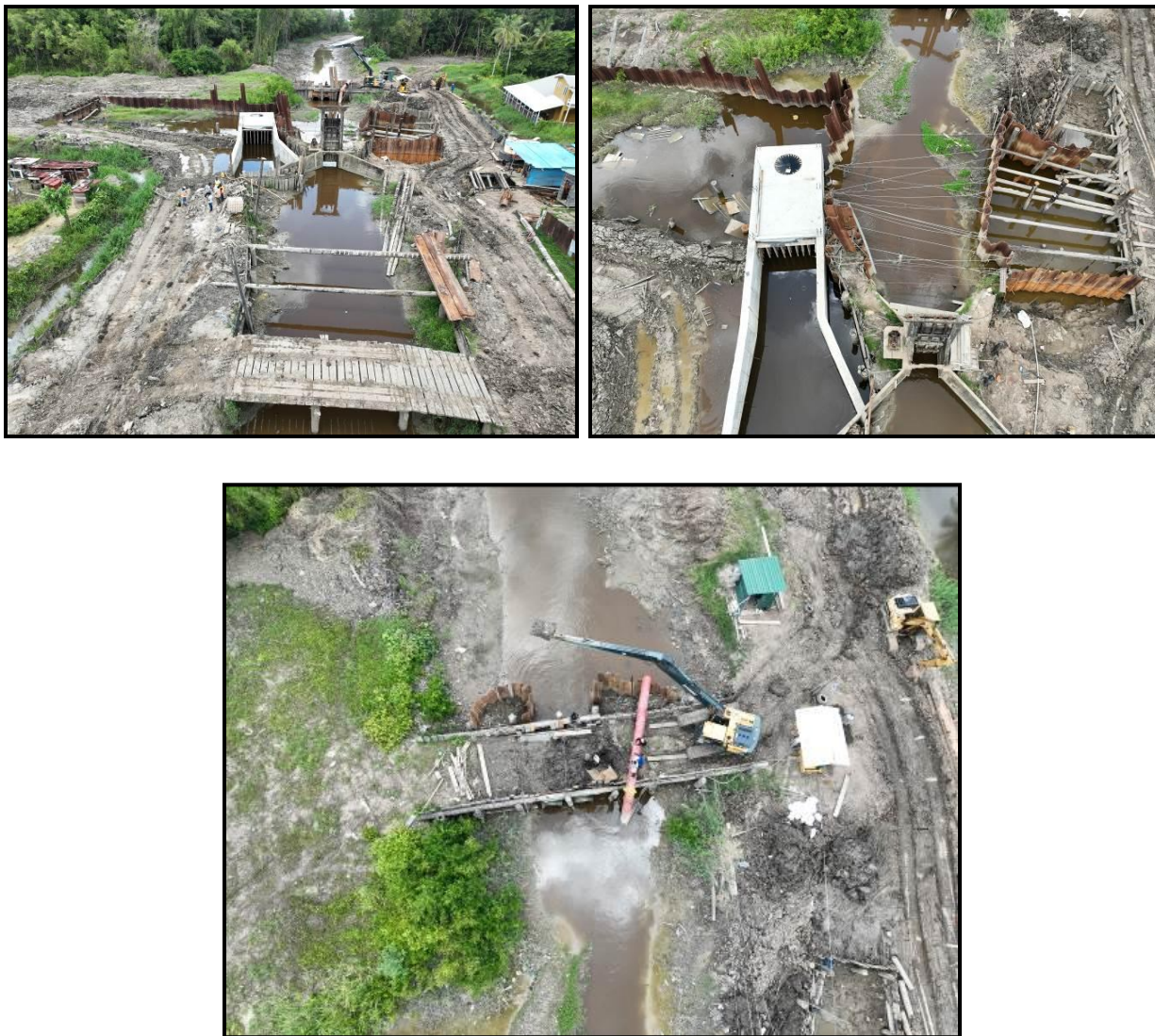
Photographs of the ongoing works – 22 August 2025
