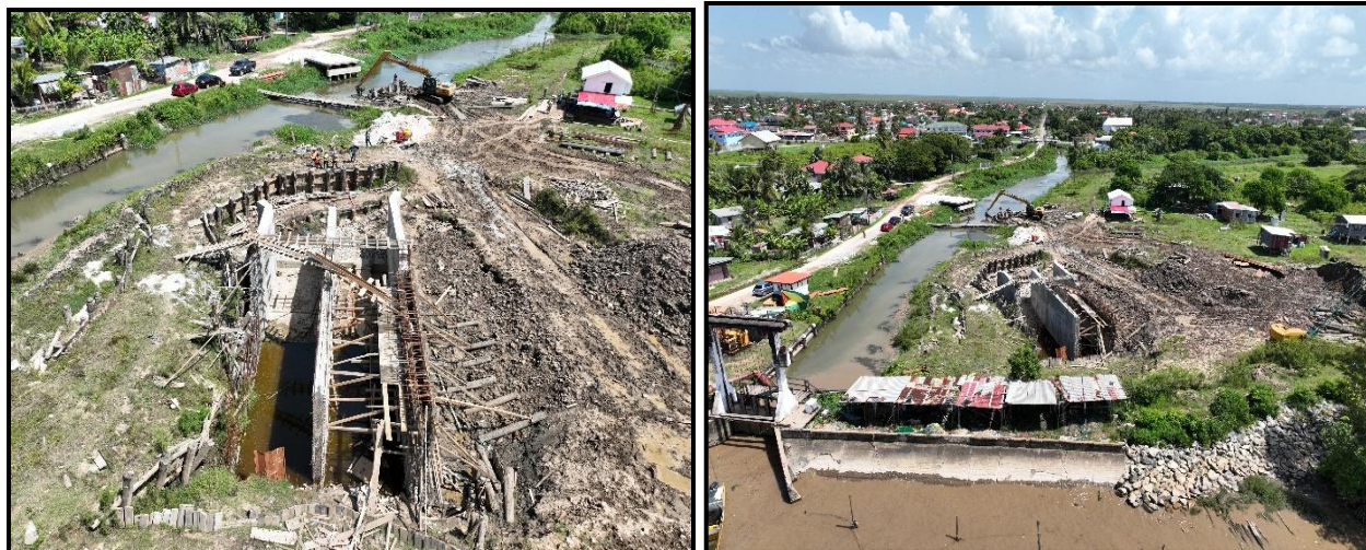
Photographs of the works in progress- 24 August 2025
